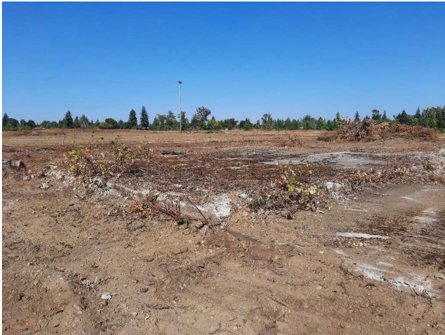
Photo 3. Overview of the project area where the plywood mill building once stood. The view is towards the northeast. Push piles visible in the midground (left and right). Photo taken September 23, 2023.
