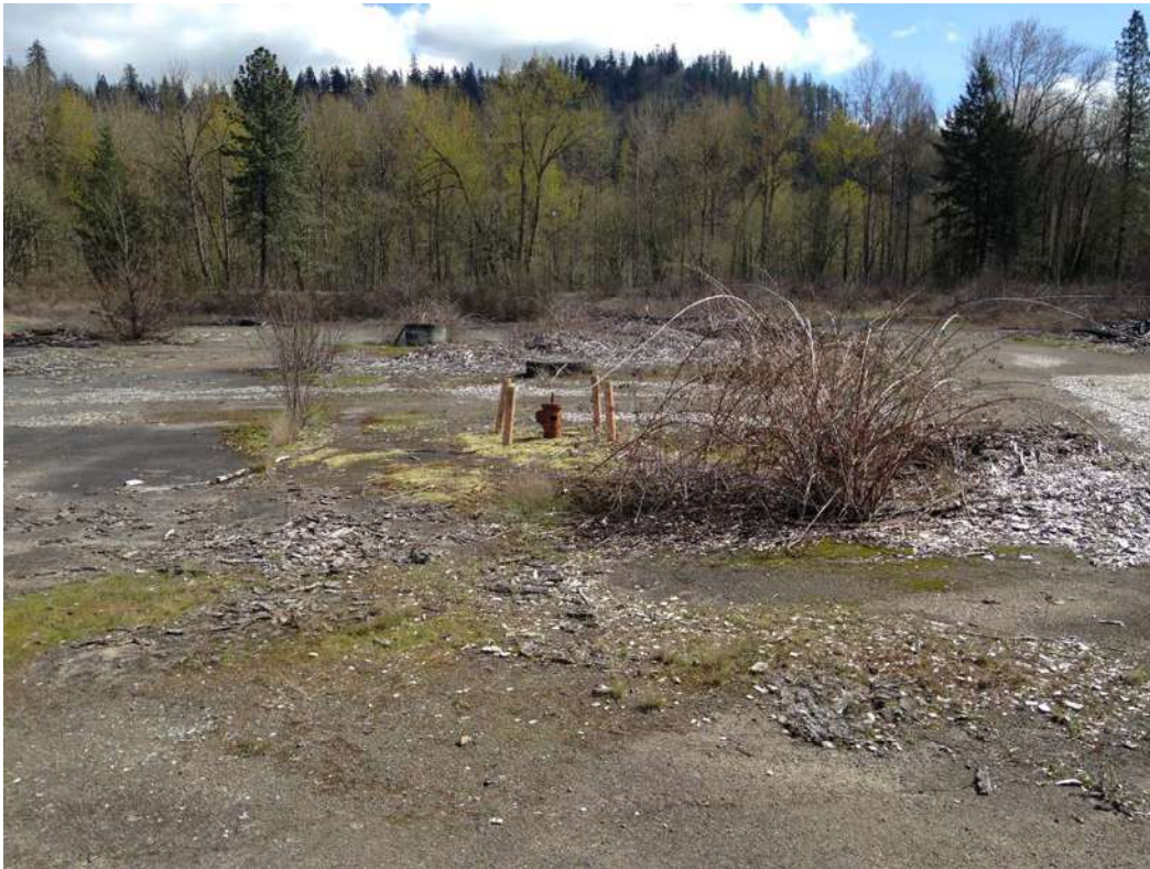
Photo 1A. Slabs and abandoned utilities looking east
