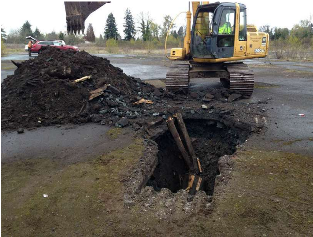
Photo 4A. Wood debris being removed from TP-3
