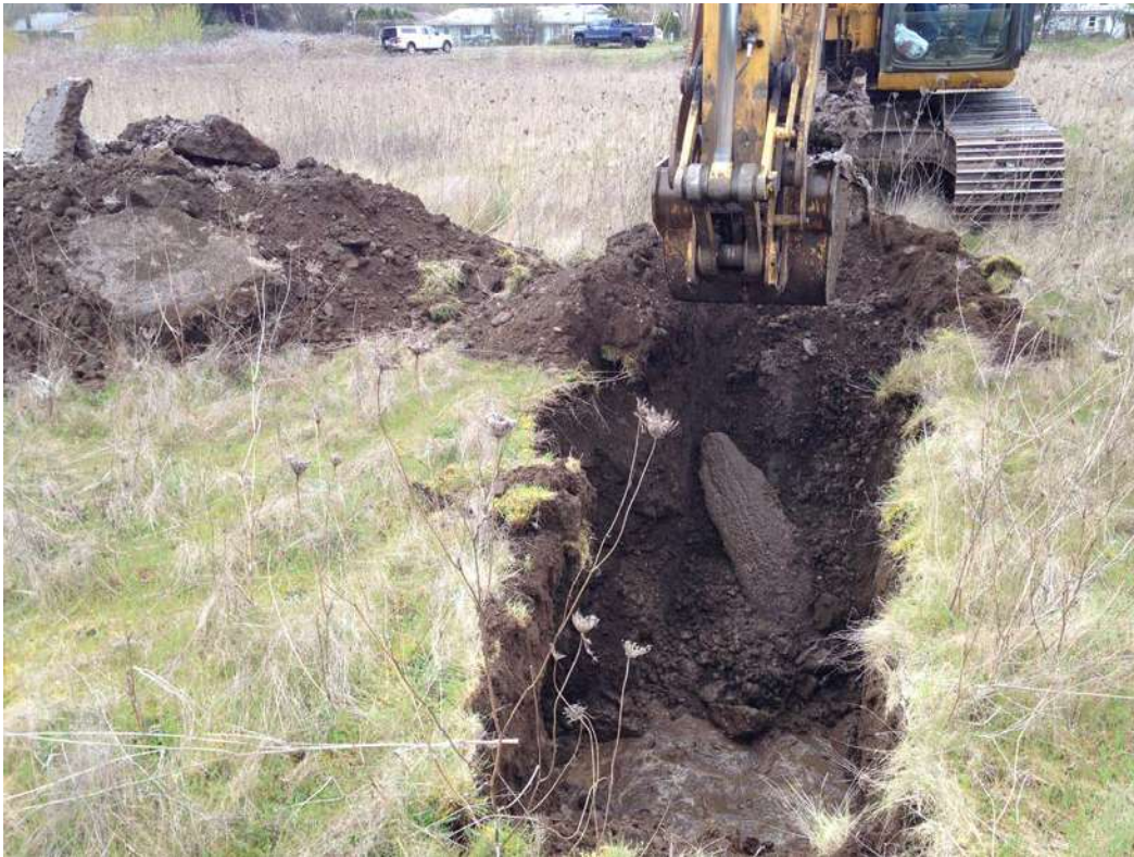
Photo 3A. Large concrete fragments being removed from TP-6
